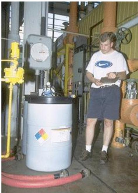
**A 55-gallon drum of phosphoric acid with proper labeling, including the manufacturer's label, and NFPA 704 hazard placard.**
